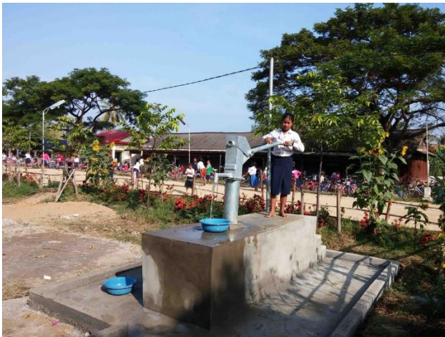
FIGURE 2: FLOOD-PROOF (RAISED) WELL IN BAK AMREK PRIMARY SCHOOL, BATTAMBANG PROVINCE, © CCCA, 2013
